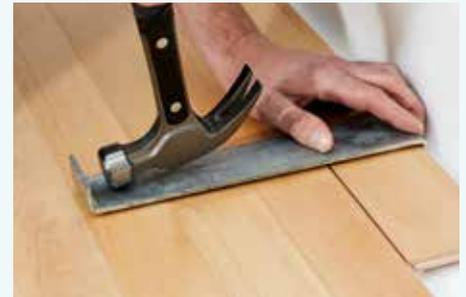
**8c** Use a joint puller to slot the last floor board into place.
