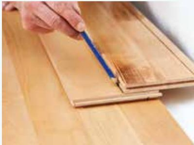
**08** **8a** The last row of boards must be trimmed to width. Remember to leave the clear expansion gap between the board and the wall.
