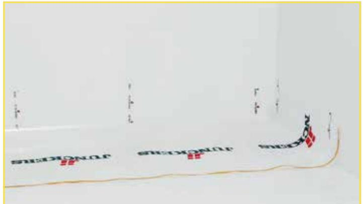
**02** On concrete and screeded floors use Junckers PolyFoam as a combined underlay and moisture barrier, with lapped joints and turned well up at walls, etc. Remember to use the built-in tape to join the overlaps.
