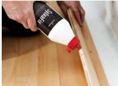
**8b** The tongue of floor boards in last row are glued and assembled to the floor boards in previous row. Only the last row floor boards are allowed to be glued lengthwise.
