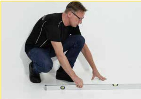
**01** Traditional straight edge: The subfloor must be flat with a maximum deviation of 2mm under a 1.5 m straight edge (UK: 3mm under a 2 m straight edge). The surface must be smooth. Any minor irregularities must be corrected.
